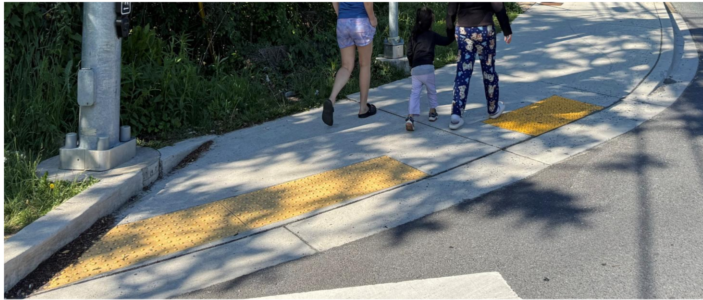
Curb ramp lacks grade separation at Glenallan Avenue and Randolph Road.
