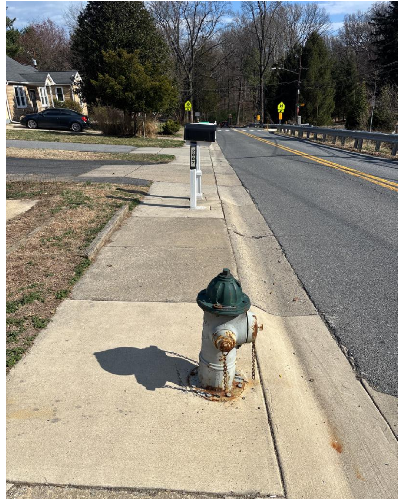
Glenallan Avenue sidewalk with utility and mailbox obstructions.
