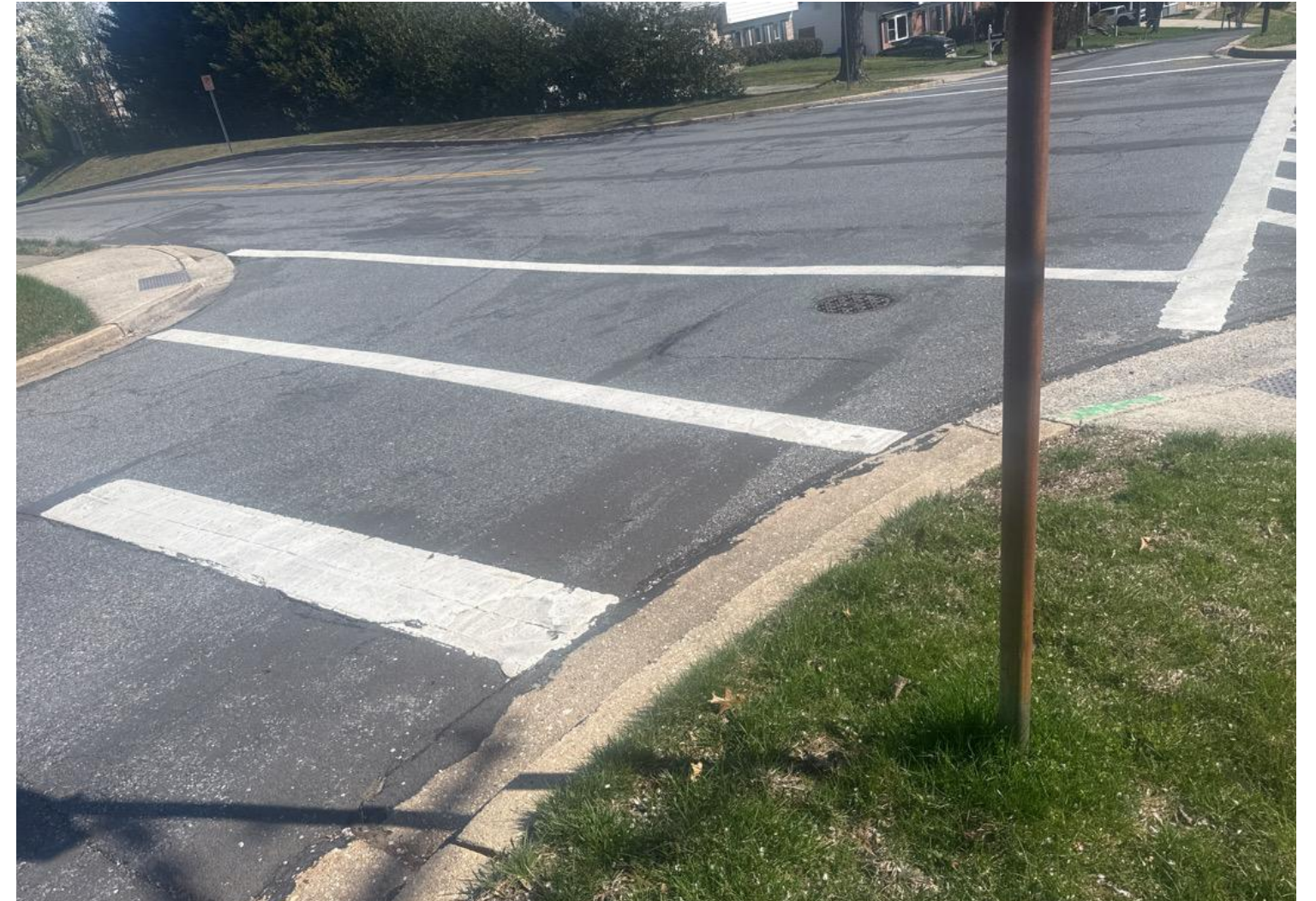
Crosswalk at Billman Lane and Garden Gate Road is not high-visibility.
