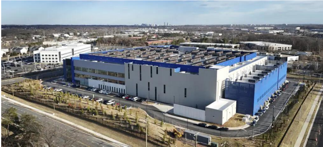
Source: Vantage Data Centers, Ashburn II Data Center Campus
