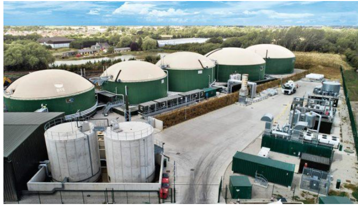
BTS anaerobic digestion system at the Maryland Food Center in Jessup, Maryland. – (courtesy BioCycle)
