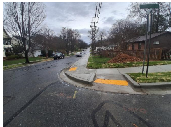
Figure 6 - New sidewalk ramps installed as concrete construction underway for McComas Avenue Neighborhood Greenway with repaving and traffic calming measures to be installed spring 2026.
