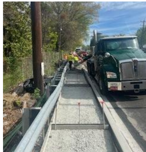
Figure 5 - Construction workers laying concrete as part of New Hampshire Avenue safety project .
