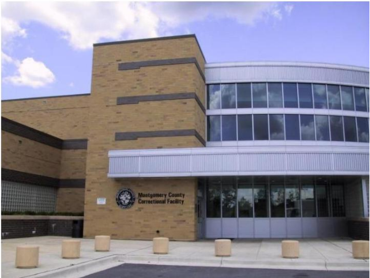
Figure 3: Front exterior of the Montgomery County Correctional Facility with brick walls, curved glass window section, and entrance area with bollards.
