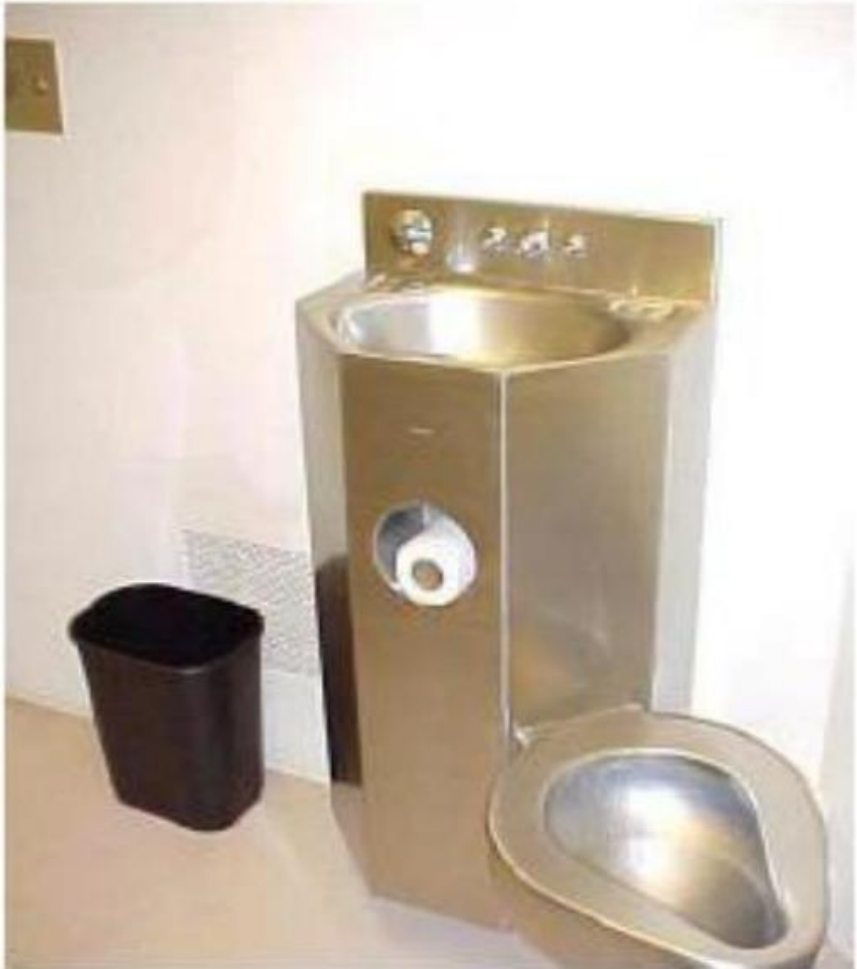
Figure 6: Example of a toilet and sink combination unit that is free of debris, with all surfaces clear and a trash bag shown without a trash bag liner, as required.
