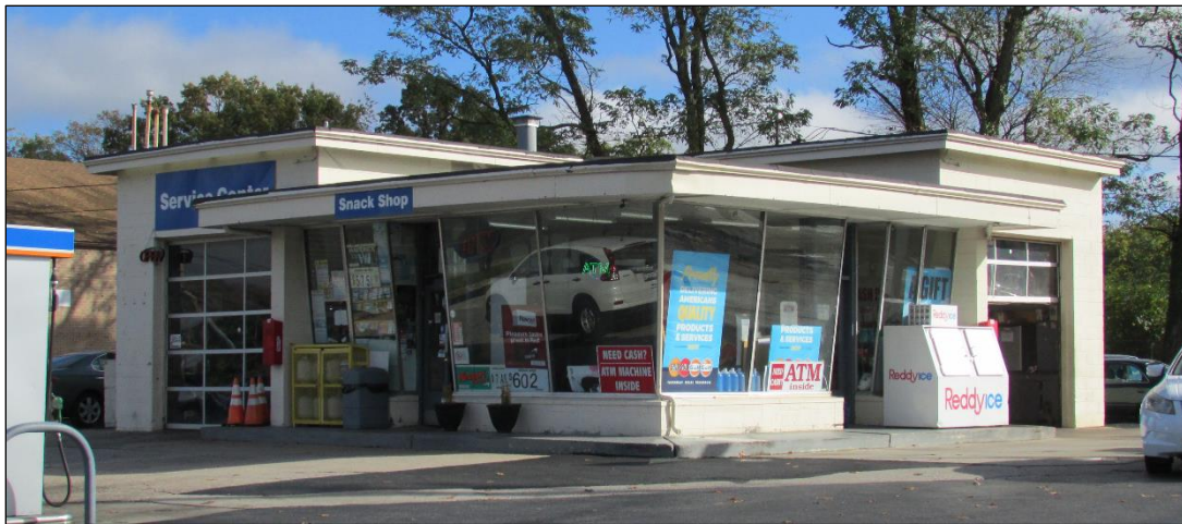
Figure 8-9: Phillips Service Station (M: 26-68), Southwest Oblique.
