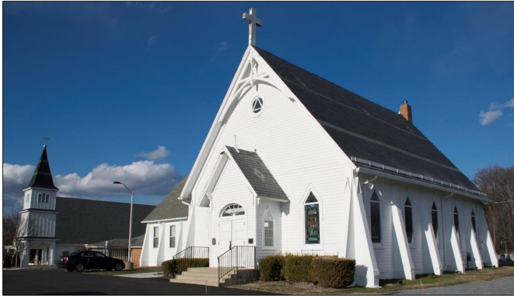
Figure 8-29: Neelsville Presbyterian Church (M: 19-5), Looking Northeast.
